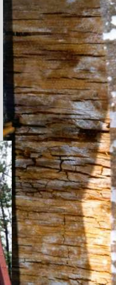
Above: the decayed sheathing was under the siding.
