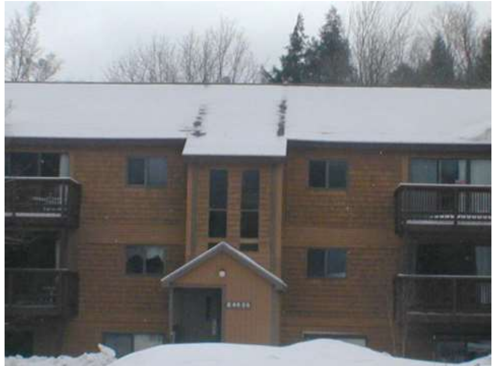
Masonry fire wall pattern
