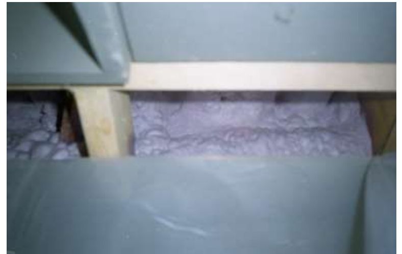
After air sealing
