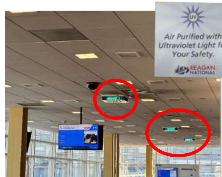
GUV fixtures in gate areas of Reagan National and Dulles airports in Washington, D.C.
